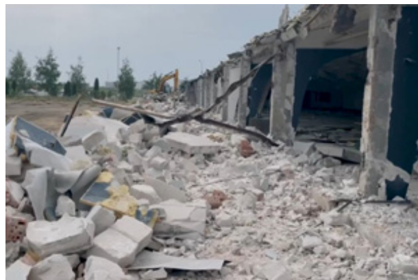
Destruction of the New Life Church building. Photo: New Life Church
